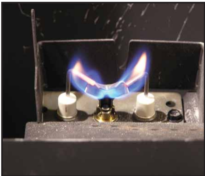
Figure 3.1 IPI Pilot Flame Patterns
