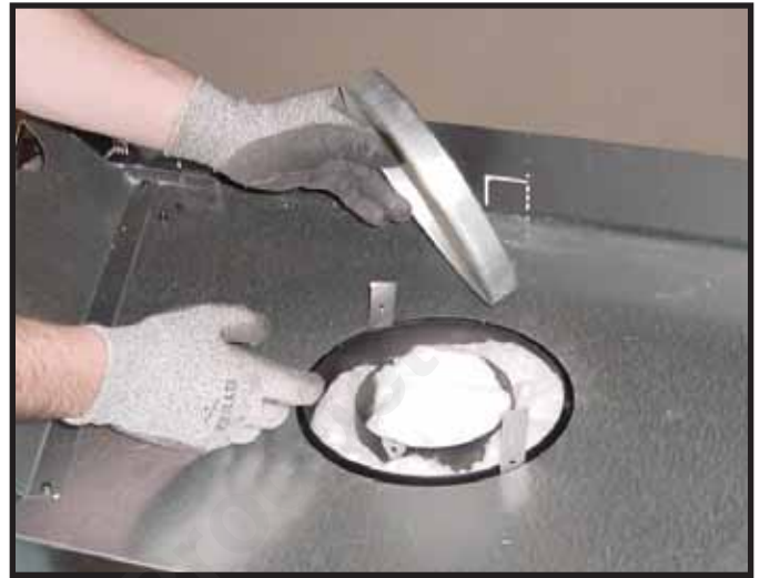
Figure 9.4 Remove the seal cap.
