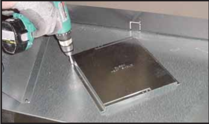
Figure 9.1 For top vent, remove the two screws holding the elbow heat shield in place. Use this heat shield over the first elbow if applicable. For rear vent skip this step.
