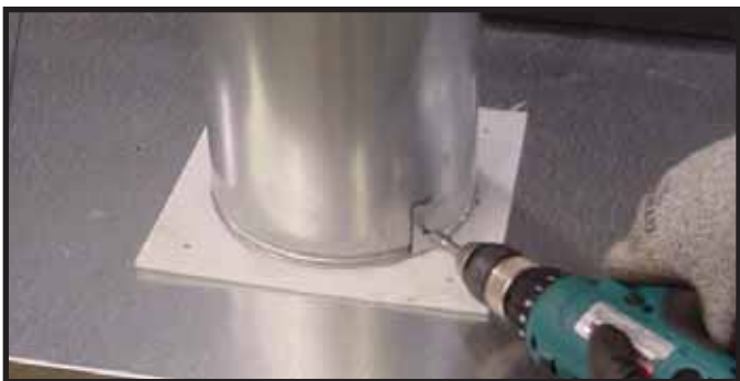
Figure 9.7 To attach the first section of vent pipe, make sure to use the fiberglass gasket in the manual bag to seal between the first vent component and the outer fireplace wrap. Use 2 self tapping screws to secure the gasket to the outer wrap.
