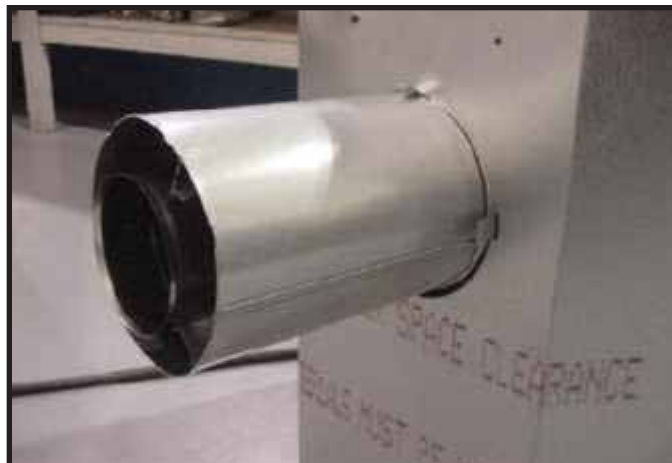
Figure 9.12 Attach the first vent section (it will snap into place). Slide the insulation gasket onto the vent section, up against the appliance and over the tabs.
