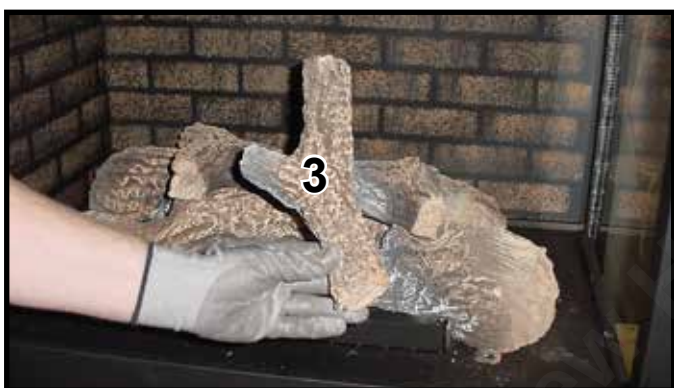
Figure 13. Placement of Log #3
