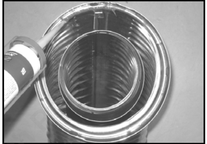
Figure 7.1 High Temperature Silicone Sealant
