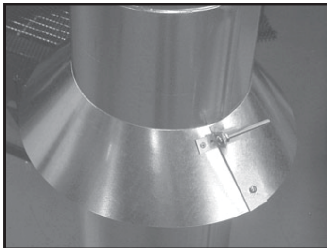
Figure 8.17 Assembling the Storm Collar Around the Pipe
