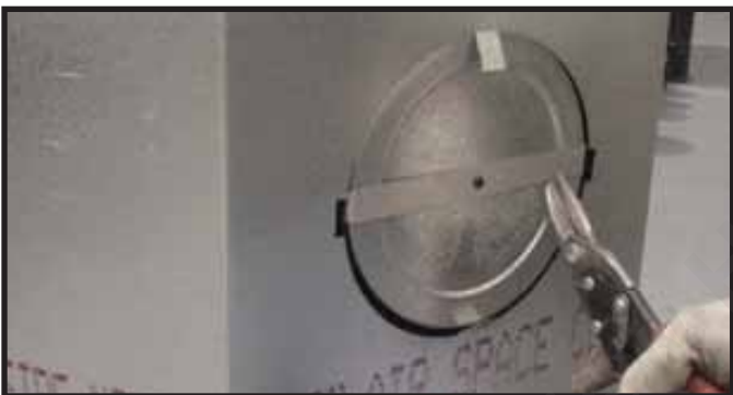
Figure 6.8 Cut the metal retaining band and fold the sides out.
