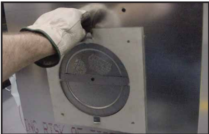
Figure 6.7 Fold the tabs toward the center of the fire plug (90°) and remove the insulation gasket.
