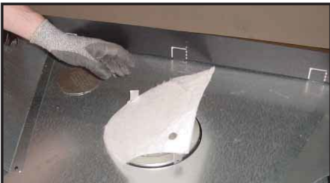
Figure 7.3 Remove the white gasket material covering the seal cap.
