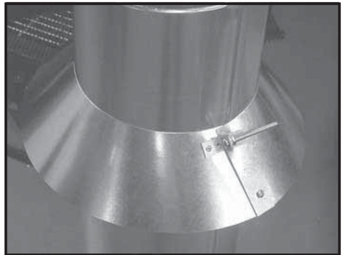
Figure 8.20 Assembling the Storm Collar Around the Pipe
