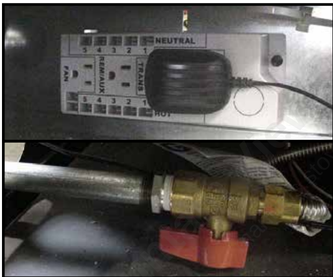
Figure 13.1 Preparation to Install Splatter Guard
