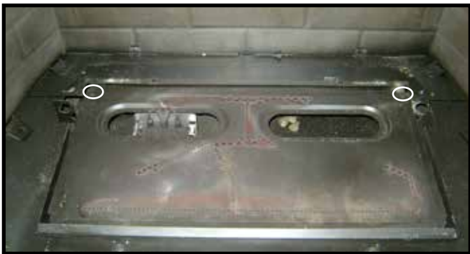
Figure 4.9 Remove Screws from Burner Assembly Rear Corners
