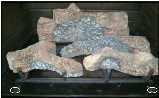
Figure 4.4 Remove Screws from Front Tab
