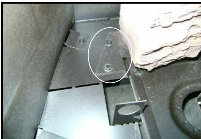
Figure 4.5 Remove Screws from Log Tabs
