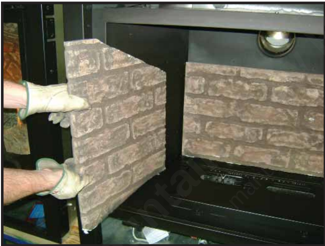
Figure 3.3 Side Refractory Removal
