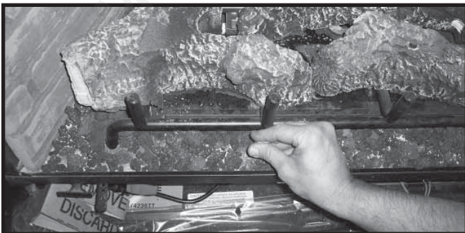
Figure 14.4 Placement of Vermiculite
