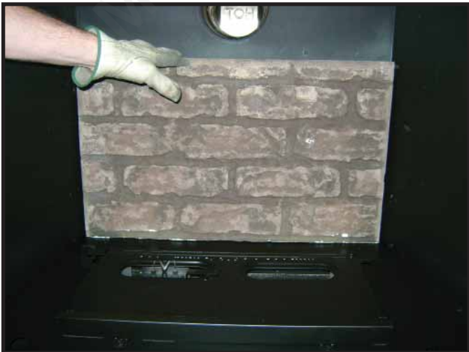
Figure 3.4 Back Refractory Removal
