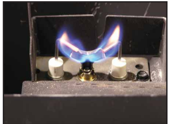
Figure 3.1 IPI Pilot Flame Patterns
