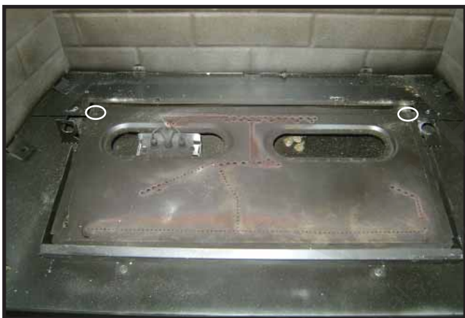
Figure 3.8 Remove Screws from Burner Assembly Rear Corners
