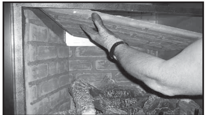
Figure 7.10 Remove Top Refractory
