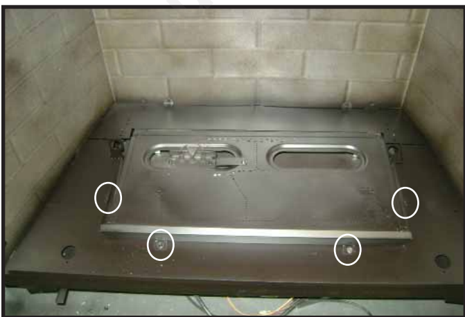
Figure 3.9 Remove Burner Skirt
