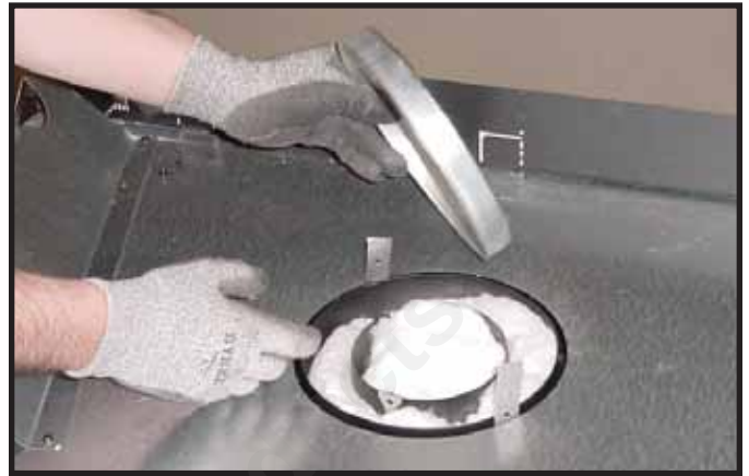
Figure 9.3 Remove the seal cap.
