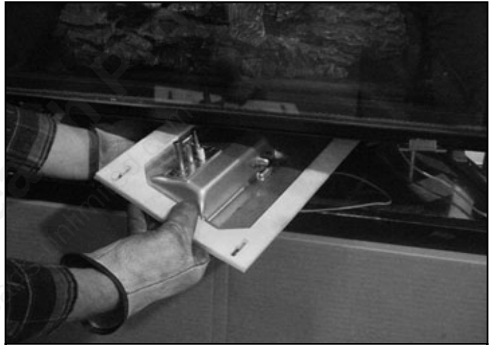
Figure 12.11 Valve Assembly
