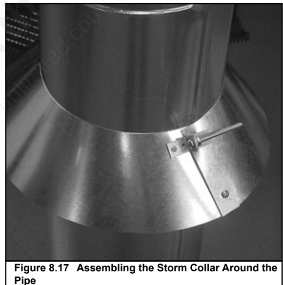
Figure 8.16 Assembling the Storm Collar
