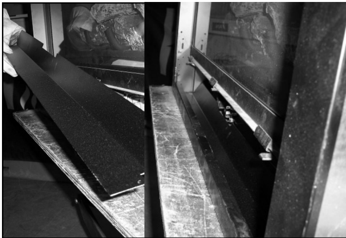
Figure 12.7 Installing Floor Cover
