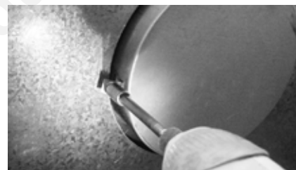
Step 5: Bend tabs out on round flue cover. Secure the round flue cover (provided) to the wrapper over the rear venting outlet. Use two (2) 3/4" long sheet metal screws
