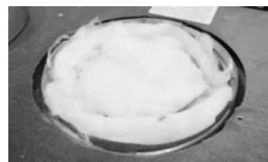
Step 3: Remove insulation from inside flue pipe.
