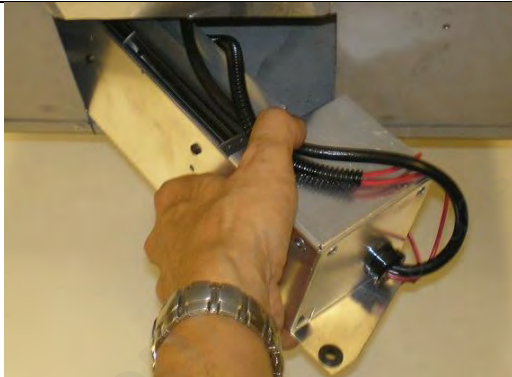
Slide Z46FK Fan Kit into opening.
