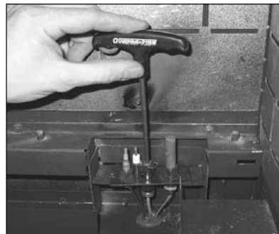
Figure 6.4 Use a 5/32" Allen wrench to remove the pilot injector.
