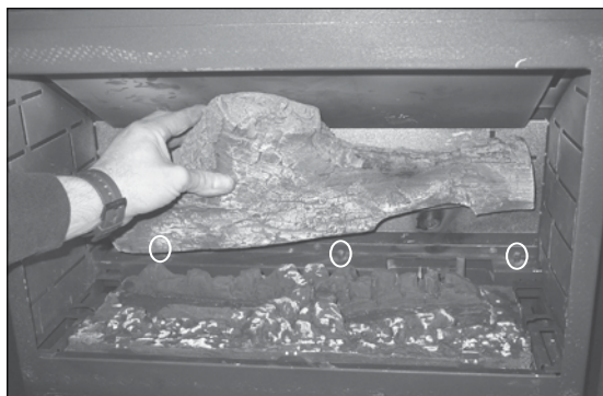
Figure 8.19 Set the rear log on the three locator pins in the back of the firebox.
