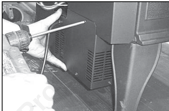
Figure 8.22 Mount blower to rear of the appliance using two screws.
