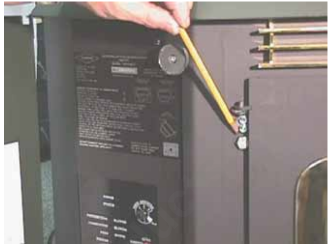
Fig.15: Draft Meter bolt hole location
