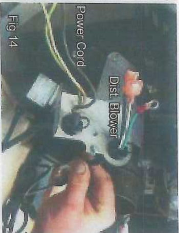
Install power cord and distribution blower cord in the cord clamp plate as shown
