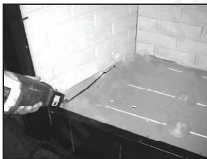
Figure 12.2. Using a saws-all, cut out the floor.
