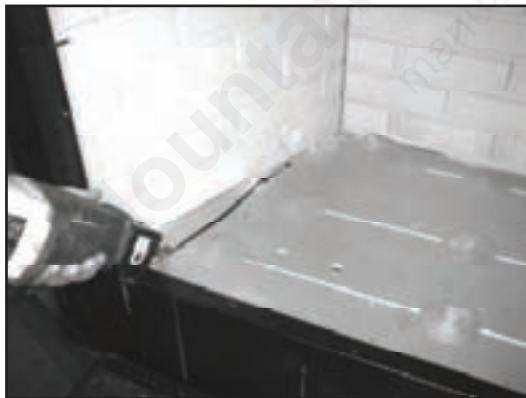
Figure 11.2. Using a saws-all, cut out the floor
