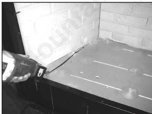
Figure 10.2. Using a saws-all, cut out the floor.
