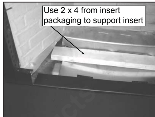
Figure 10.3. If the floor is made of thin metal, we recommend using the 2 x 4 from the insert packaging to support the insert. The 2 x 4 may need to be cut to the appropriate size.
