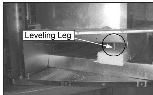
Figure 10.5. Ensure that the leveling leg is positioned over the 2 x 4 before leveling the insert.
