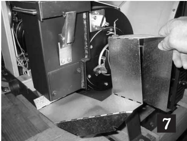
Remove blower heat shield (large inserts)
