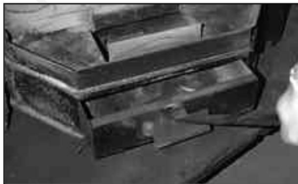
(Figure 9) - Emptying Small Ash Pan on Insert Stove
