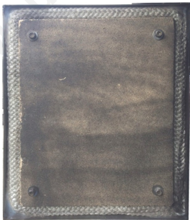
7-6-3 Completed Flue Box Door Gasket Installation
