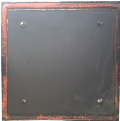
7-6-1 Completed Firebox Door Gasket Installation
