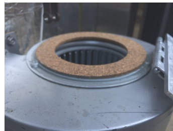
7-6-5 Completed Blower Gasket Installation
