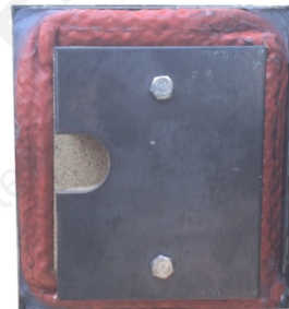
7-6-2 Completed Ash Door Gasket Installation
