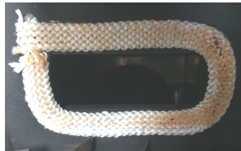
7-6-4 Completed Bypass Damper Gasket Installation
