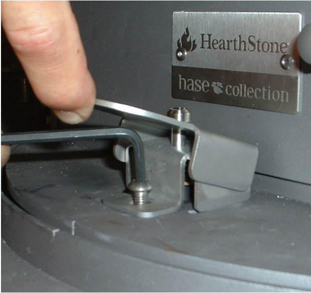
Figure 4: Remove Mounting Screw
