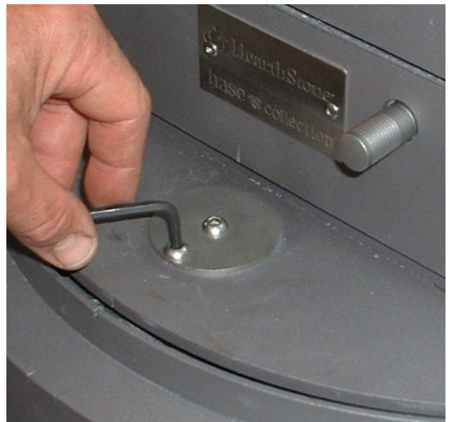
Figure 7: Tighten Mounting Screw
