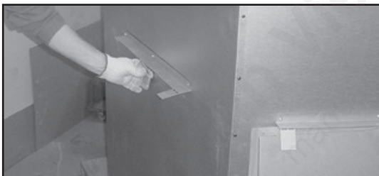
Figure 3.7 Bending Refractory Shipping Tabs Back Down
