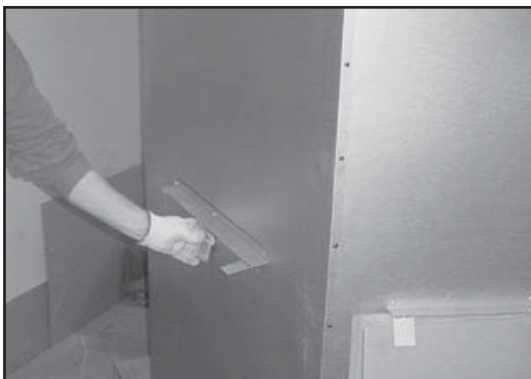
Figure 4.6 Bending Refractory Shipping Tabs Back Down
