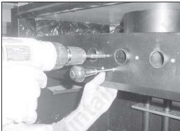
Figure 16 Line up both Seal Plates, Insulation & Smoke Shield
