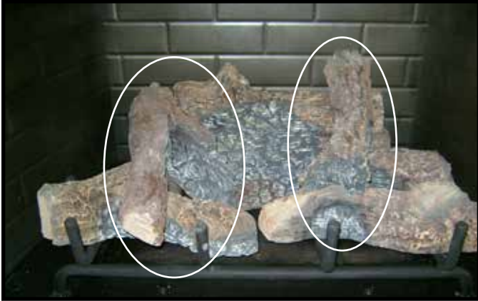
Figure 3.2 Remove Top Two Logs
