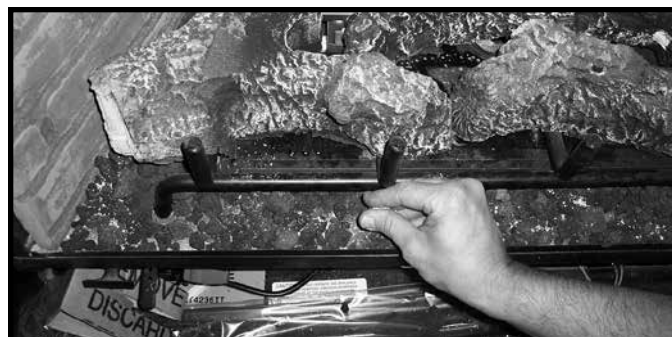
Figure 14.4 Placement of Vermiculite
