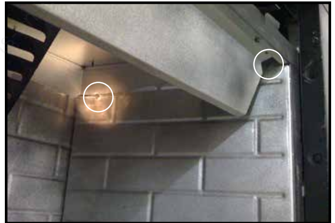
Figure 3.6 Top Screws For Metal Refractory
