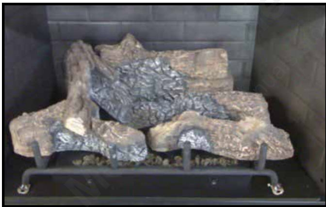
Figure 5. Left Log in Proper Position
