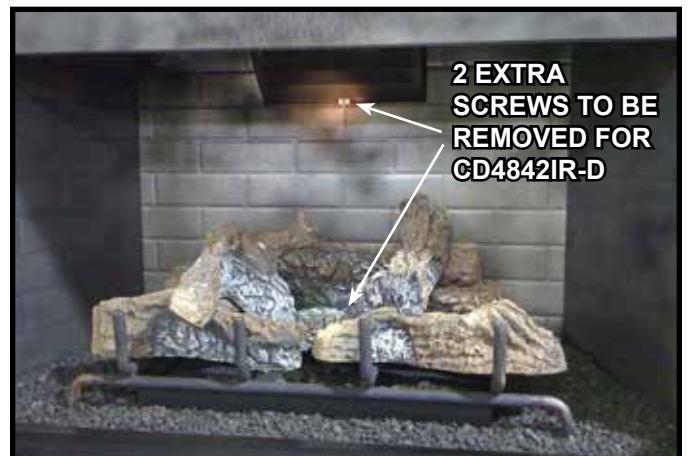
Figure 3.7 CD4842IR-D Extra Metal Refractory Screws
