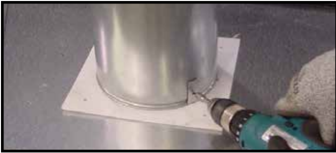
Figure 9.6 To attach the first section of vent pipe, make sure to use the fiberglass gasket in the manual bag to seal between the first vent component and the outer fireplace wrap. Use 2 self tapping screws to secure the gasket to the outer wrap.
