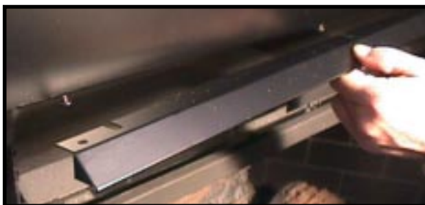
Figure 43 - Installing the Hood
