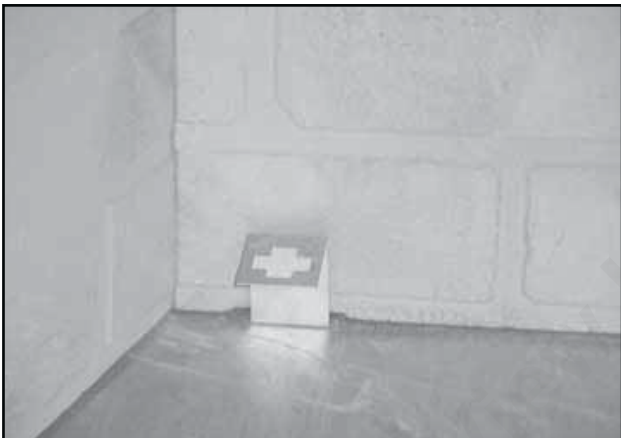
Figure 7.16 Grate Retaining Bracket in Place
