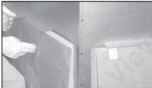
Figure 7.1 Unpack Back Refractory
