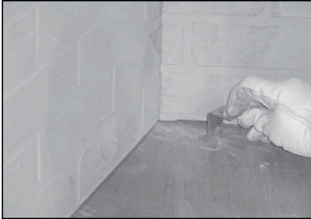
Figure 7.15 Slide Grate Retaining Bracket into Notch
