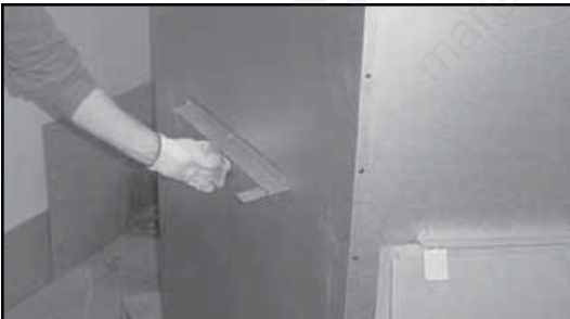
Figure 7.2 Bend Refractory Brackets Back Down
