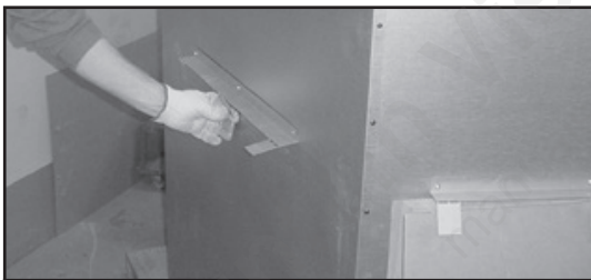
Figure 3.7 Bending Refractory Shipping Tabs Back Down
