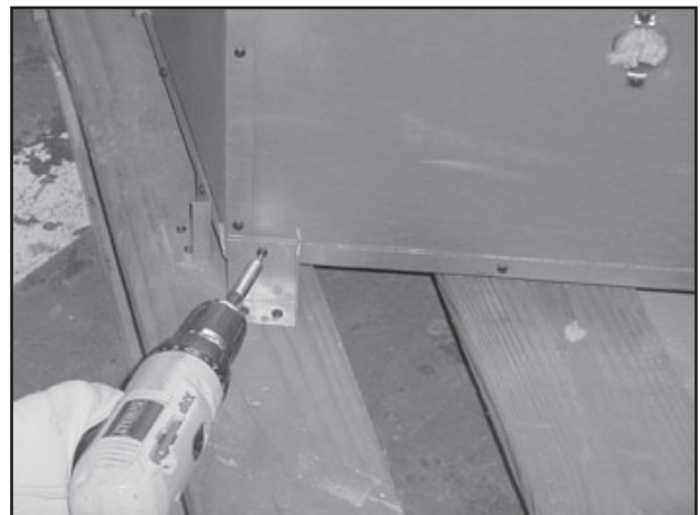
Figure 3.12 Removing Shipping Brackets
