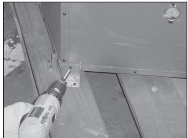
Figure 3.12 Removing Shipping Brackets
