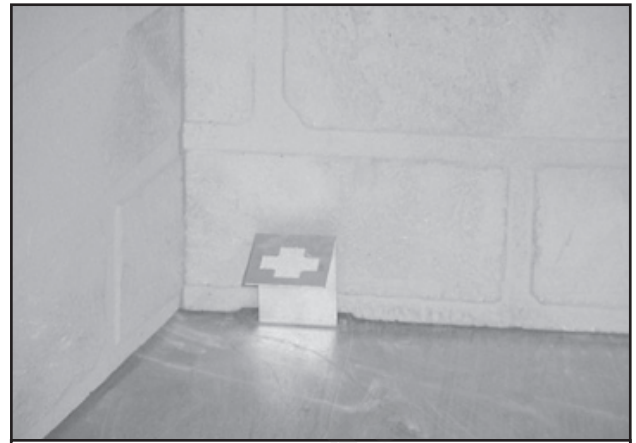
Figure 8.8 Grate Retaining Bracket in Place
