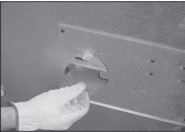
Figure 3.18 Bending Tabs on Outside Air Kit Collar
