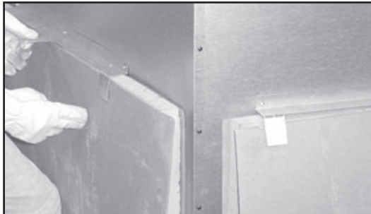
Figure 3.6 Unpack Back Refractory
