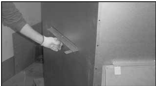
Figure 3.6 Bend Refractory Brackets Back Down
