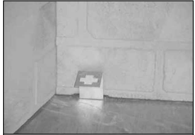
Figure 8.8 Grate Retaining Bracket in Place
