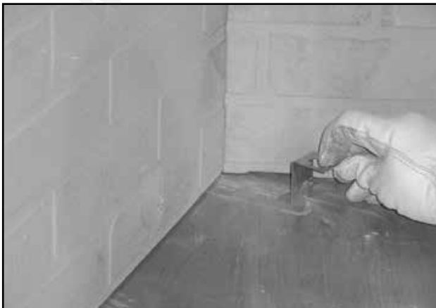
Figure 8.7 Slide Grate Retaining Bracket into Notch
