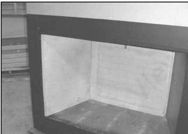
Figure 8.6 Side Refractory Installed
