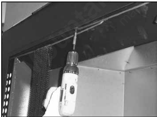
Figure 3.7 Remove Screen Rods
