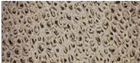
Combustor Problem - Ash, a fluffy light grey powder, and soot, accumulate on the combustor surfaces in normal use. In extreme situations combustor can become clogged and should be cleaned.
