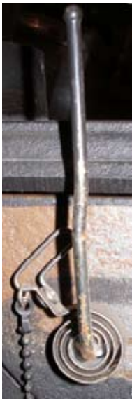
Thermostat assembly installed open position
