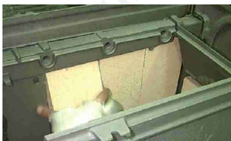
Install firebrick slim bricks
