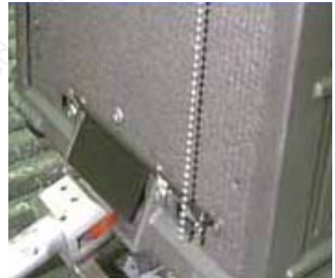
Ball chain installed using a shim
