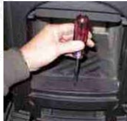
Remove primary air manifold
