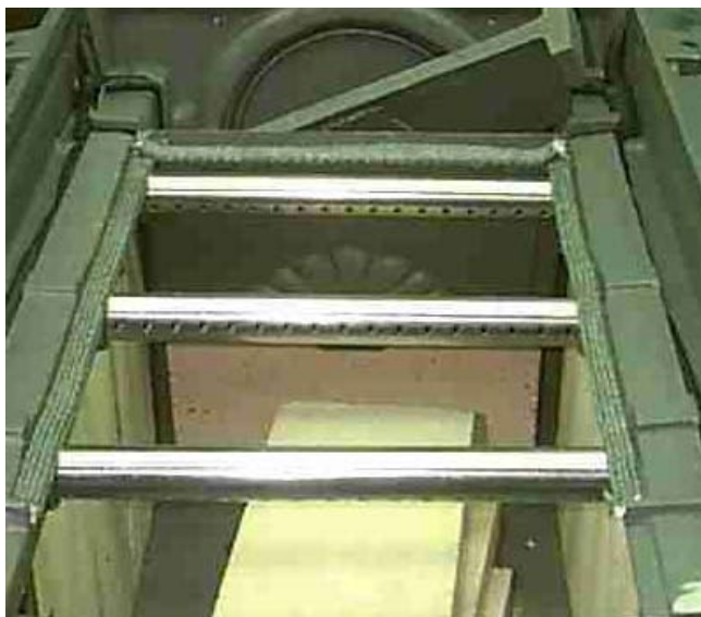
Install secondary air tubes and gasket tape
