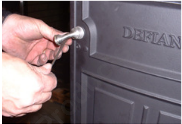
Fig. 29 Install Damper Stub
