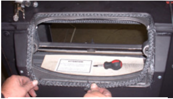
Fig. G-5 Flue Collar 7/16" x 52" Fiberglass Flue collar to top & back
