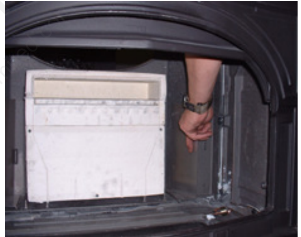
Fig. 19 Install Refractory Assembly
