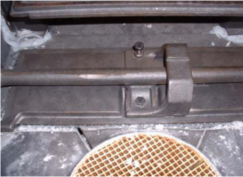
Damper in closed position with the damper crank rotated to locked on the damper ramp of the adjuster.
