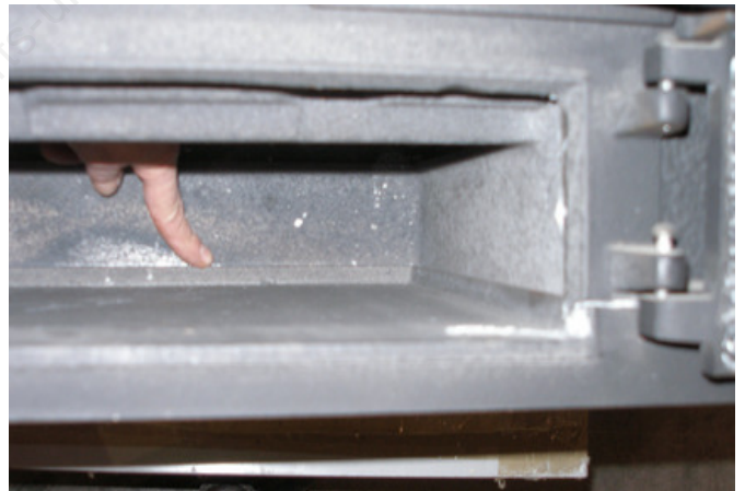
Fig. 9 Smooth out any excess cement from the cement seams
