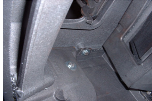
FIG. 11 Interior Top Attachent Hex Head Bolt
