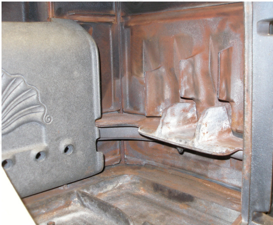
Lower Fireback in Place with Shim
