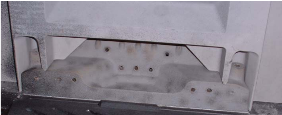
Shoe Installed in Fireback
